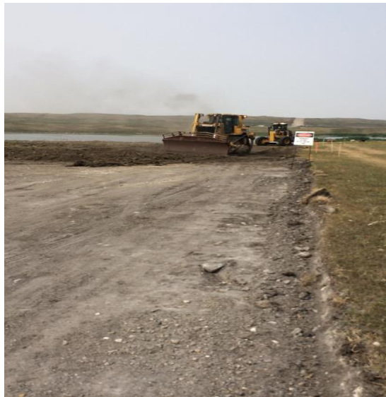
Equipment Stripped top layer to extend HDD pad to 624+700 additional 30m within Areological site.
