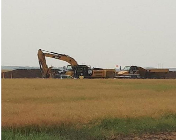
SF 58 Stripping and piling topsoil
