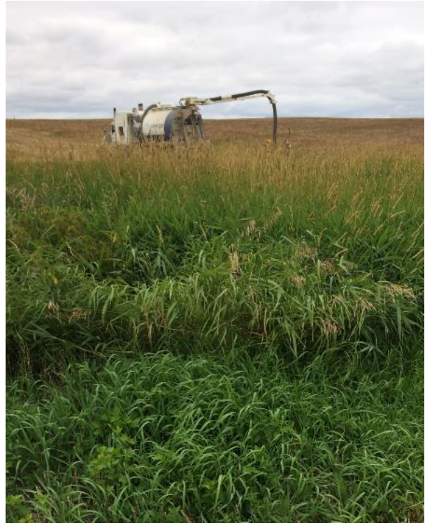
SF 63 643+400 to 643+600 hydro vac (Valley west of the old rail bed) Hydrovac to expose the pipe.
